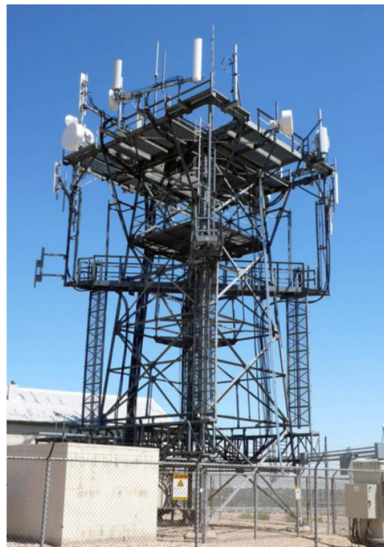
Figure 6-3: Communication Systems on Tower in Broomfield, Colorado, USA (Photo by Frank Sanders, [105, p. 15]).
